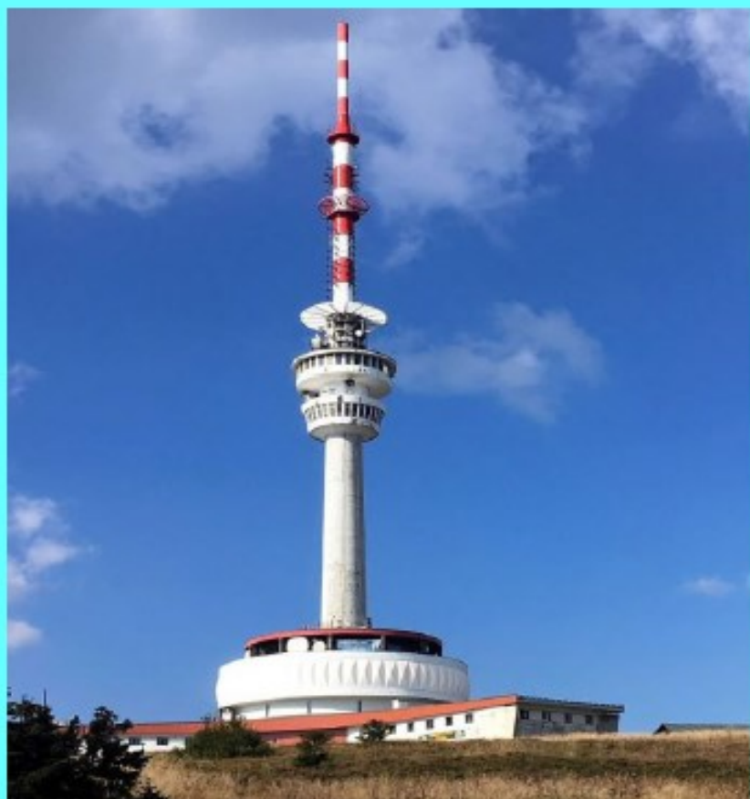
De TV zender op de locatie Praded Mountain (CZE). The TV transmitter at the location Praded Mountain (CZE). České Radiokomunikace, via Gösta van der Linden, 2022.
