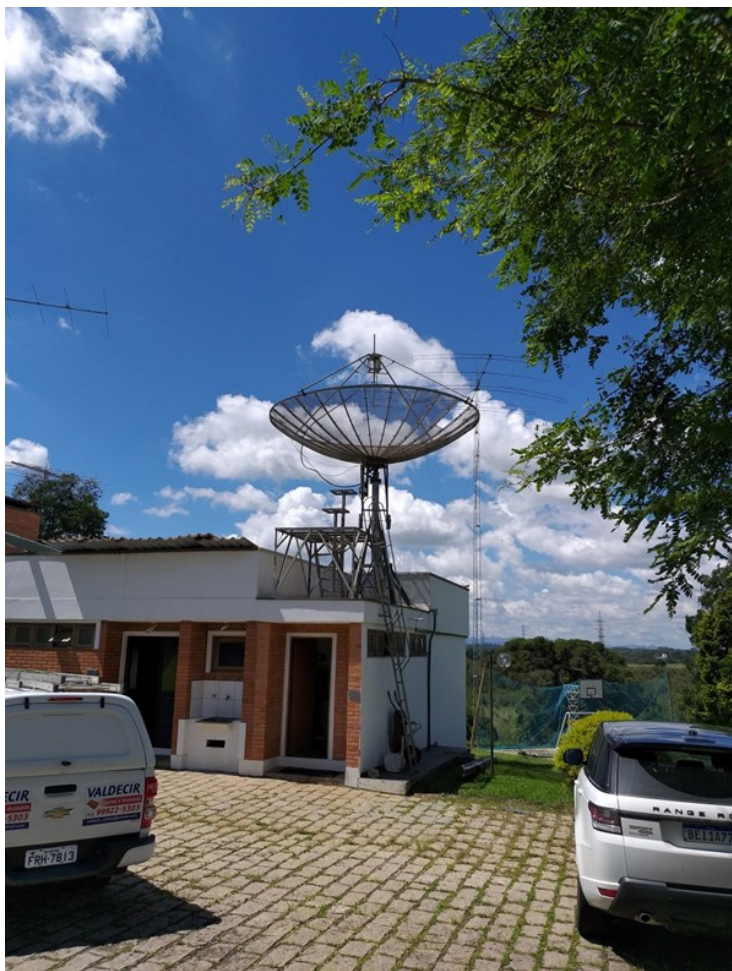
Moon Bounce Antenne (6 meter parabool - EME 144 MHz)
