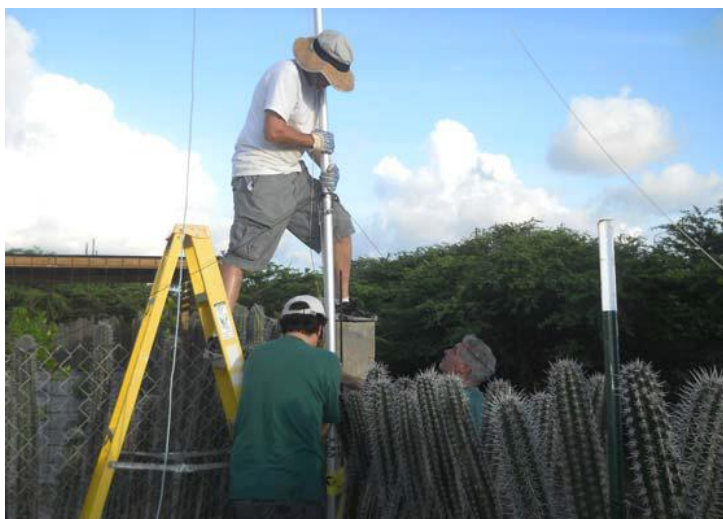
Ward, NOAX , raising a Spiderbeam on a telescopic aluminium mast at PJ4Q, November 2013. Assisting are Scott, W4PA , and (behind the cactus) Brad, WF7T . Don't lose your balance, Ward!
